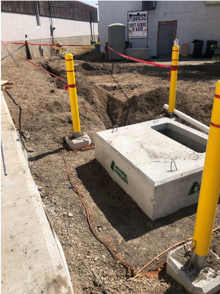
Installation of new electrical service conduits and transformer base
