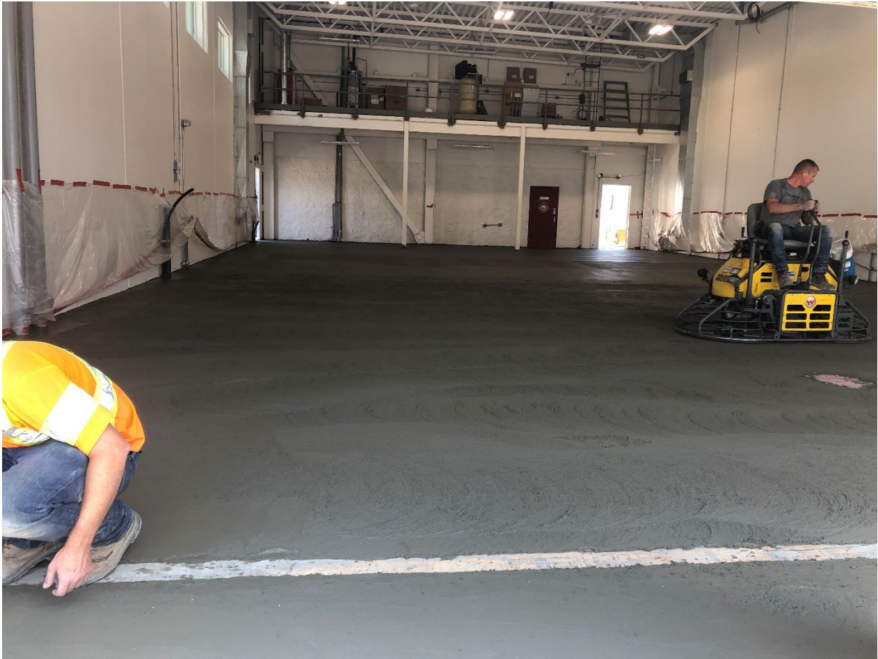
Power-troweling new concrete floor
