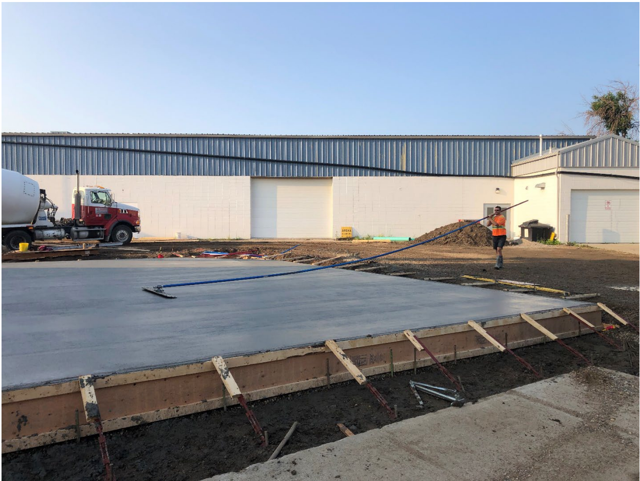
Pouring concrete on front apron
