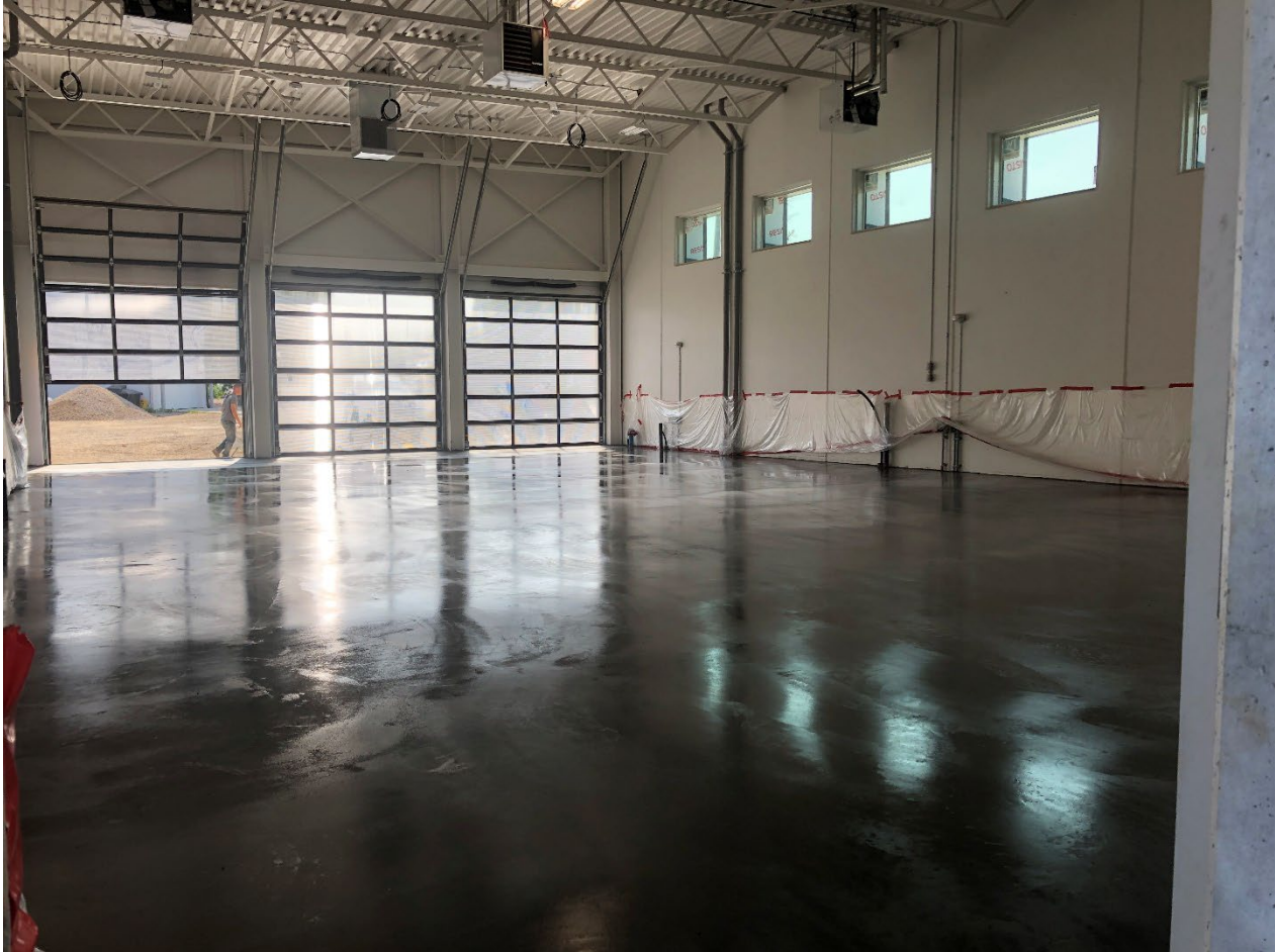
Concrete sealant applied to new floor
