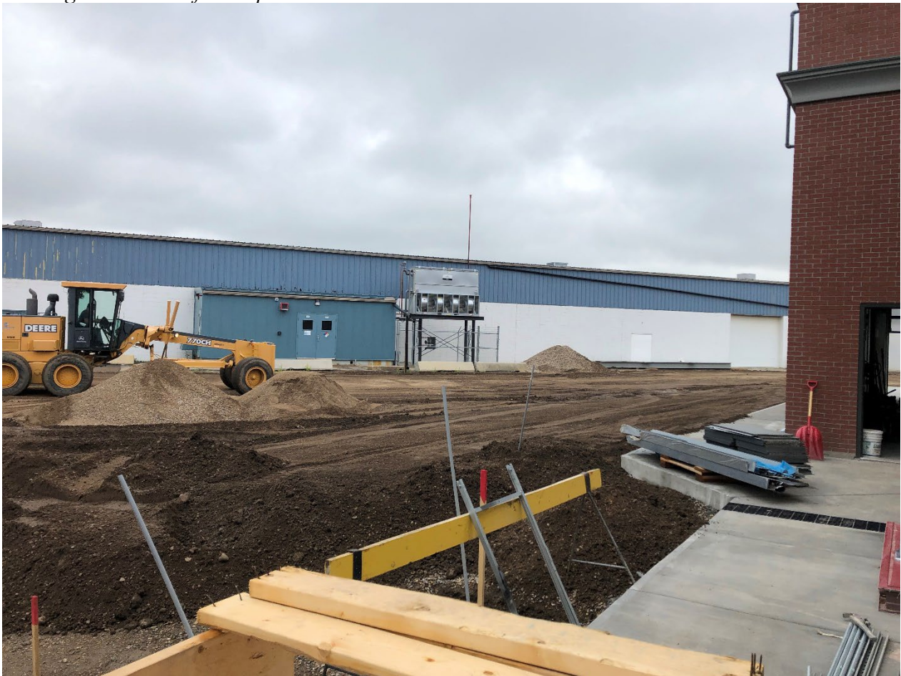
Grading of parking lot after completion of all underground services
