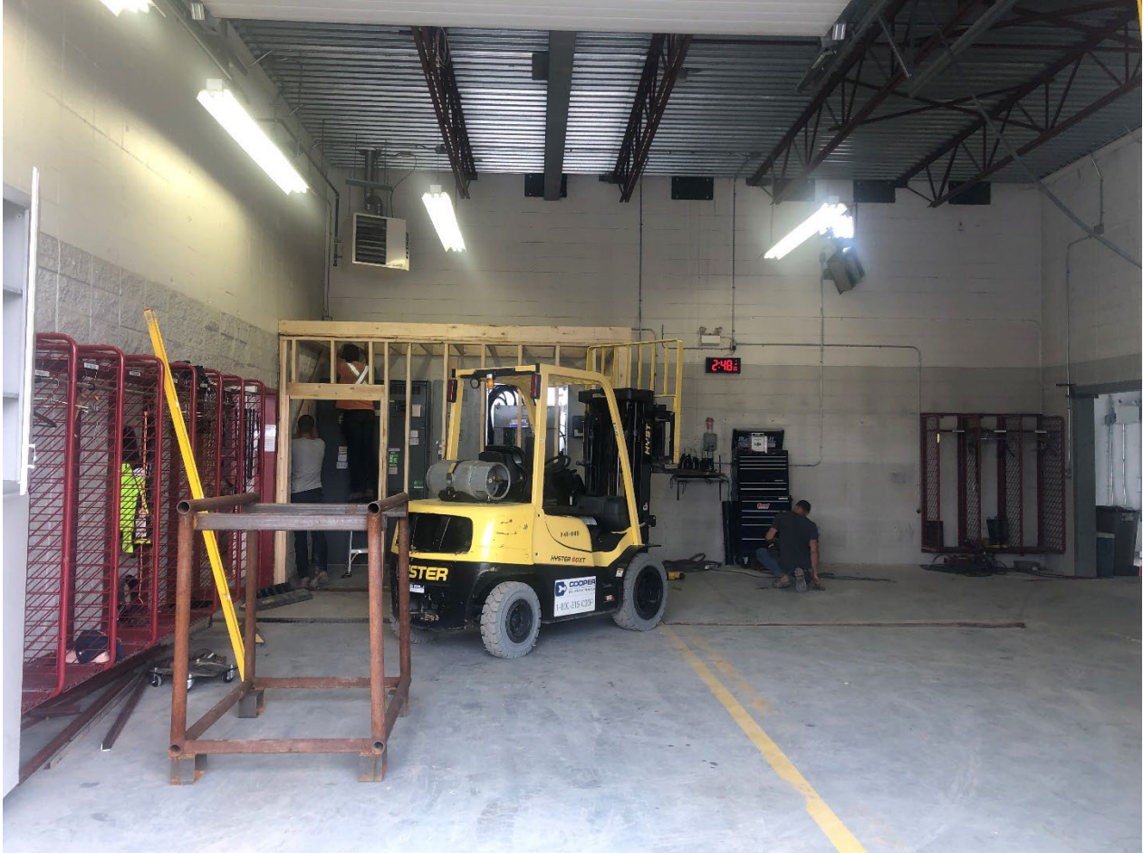
Framing of new electrical room in existing bays
