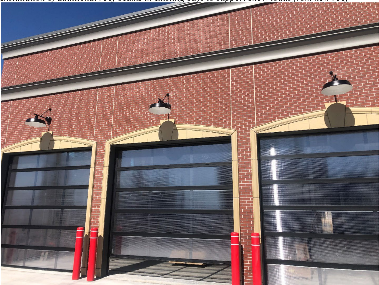
New overhead doors and exterior lights installed
