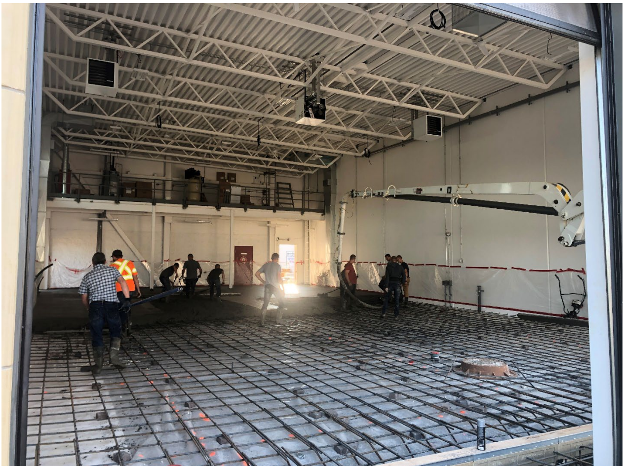
Pouring concrete floor in new bays
