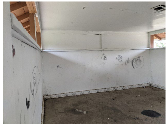
Interior Photo No. 2
