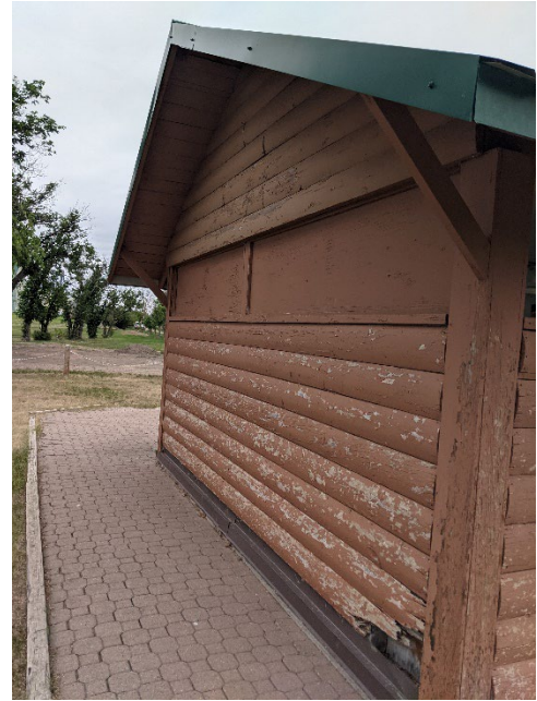
Exterior Photo No. 2
