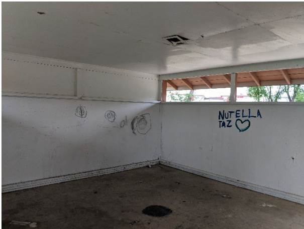
Interior Photo No. 1
