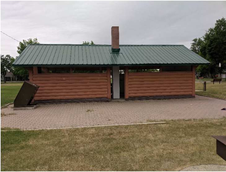
Exterior Photo No.1
