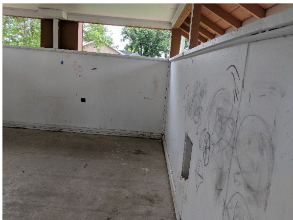
Interior Photo No. 3
