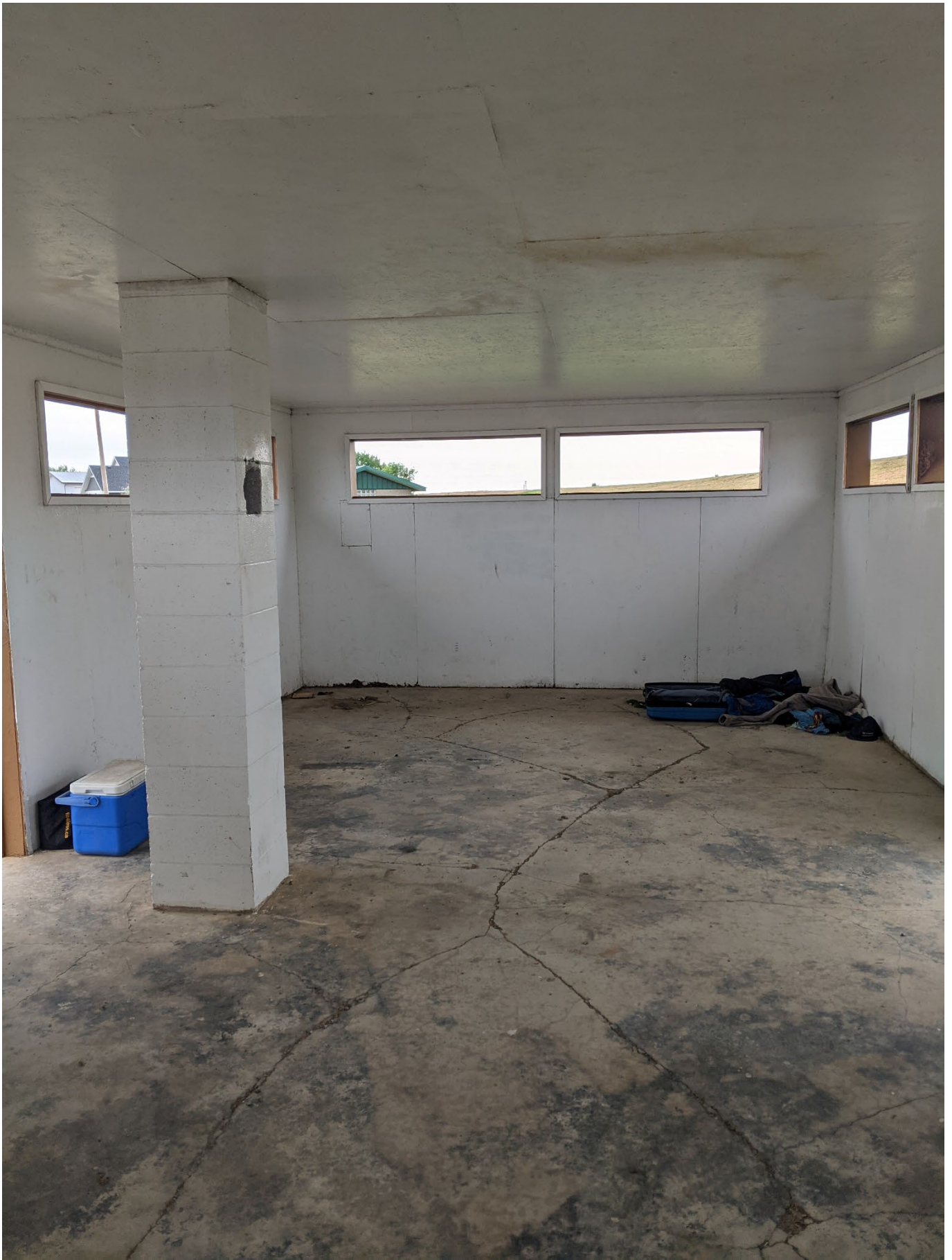
Interior photo No. 2 (Looking West)
