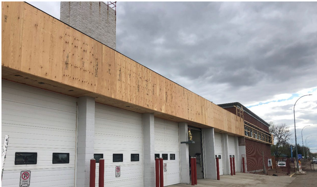
Installation of the exterior crown moulding and facade
